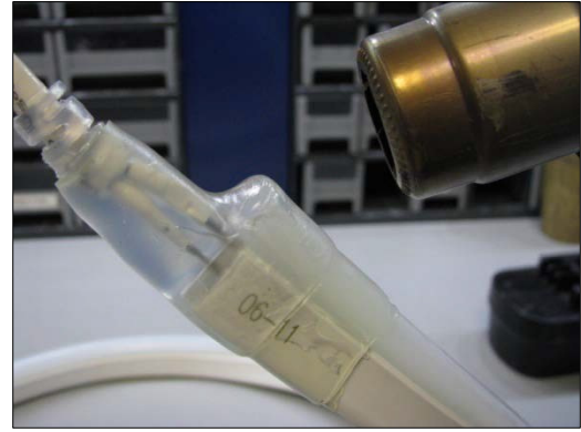
Apply heat to seal joint
