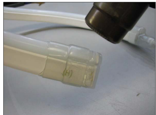
Apply heat to seal joint
