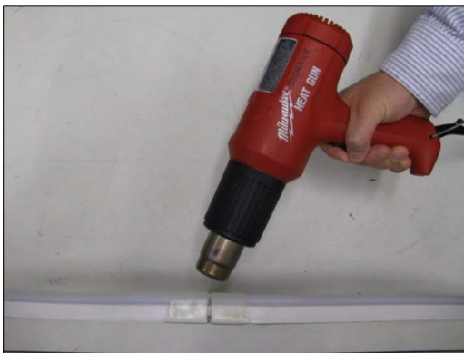
Heat shrink tubing at splice
